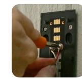
The wiring must be connected to a transformer with a voltage of 8VAC - 24VAC and an internal
